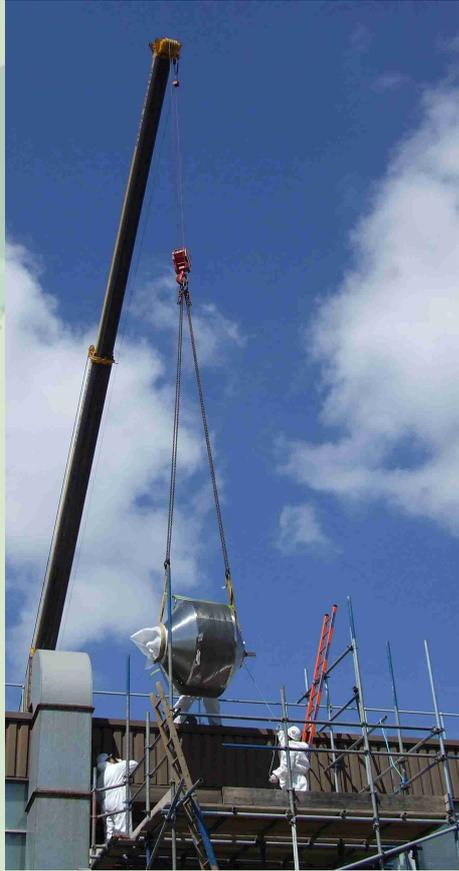
As each of the parts were carefully transferred to the platform, the task was then to move them into the room and lower them to the floor 1.2m below the window opening.
