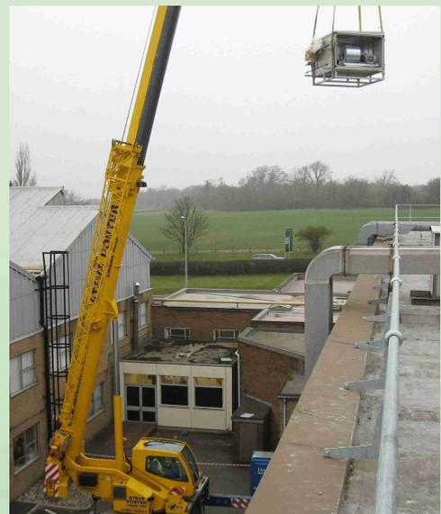
The air handling unit, extract fan and filter unit had already been placed on the roof.
