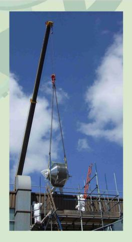
As each of the parts were carefully transferred to the platform, the task was then to move them into the room and lower them to the floor 1.2m below the window opening.
