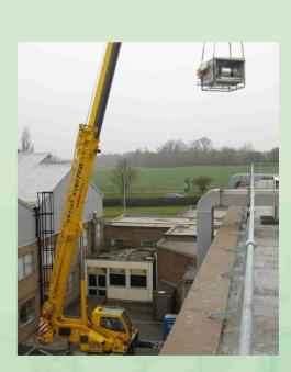
The air handling unit, extract fan and filter unit had already been placed on the roof.
